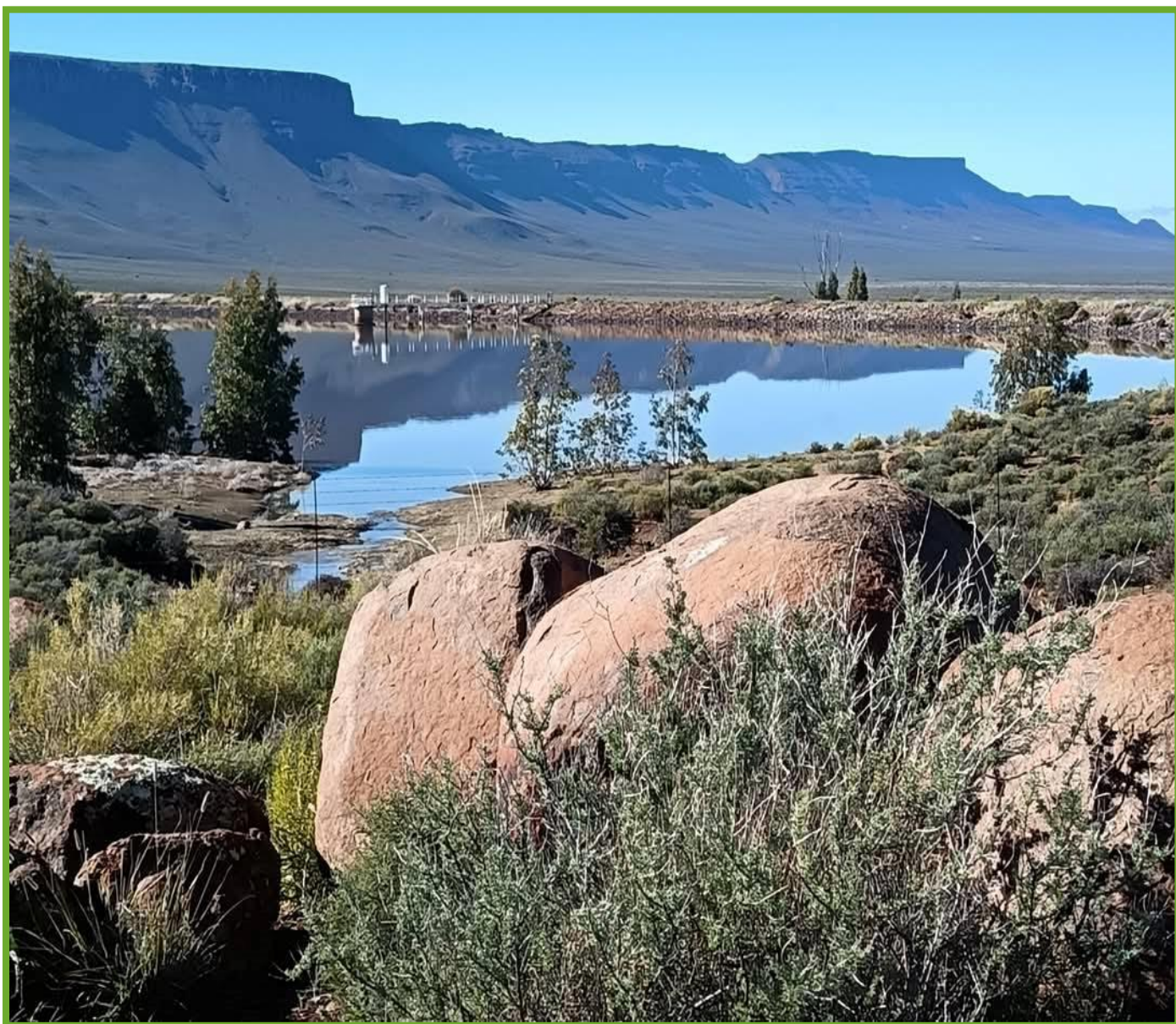
Pictures 1: Dam – water level
